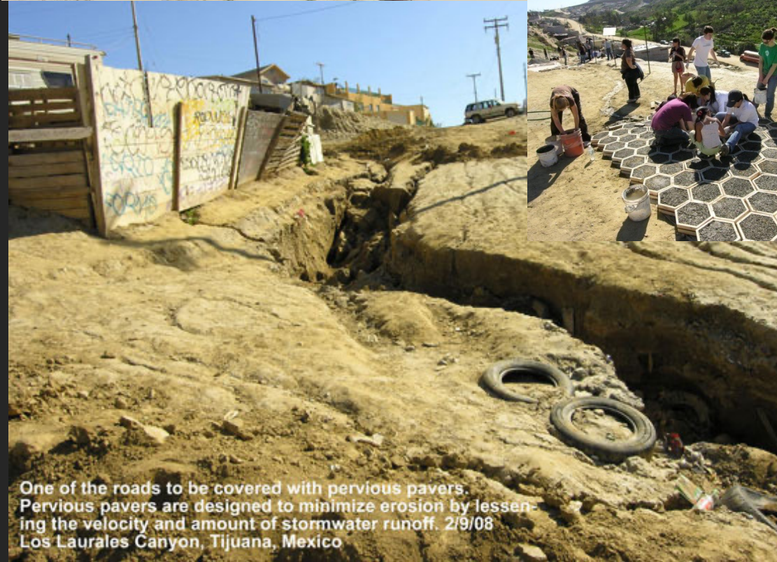
Students mixing aggregate for constructing pervious pavers
